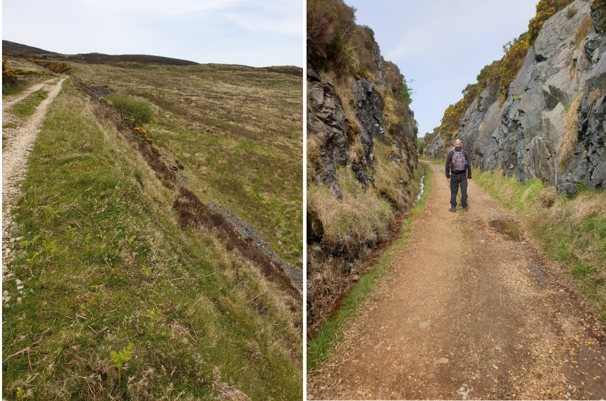
High embankment section (left) and 'canyon' section (right) (both facing west).
