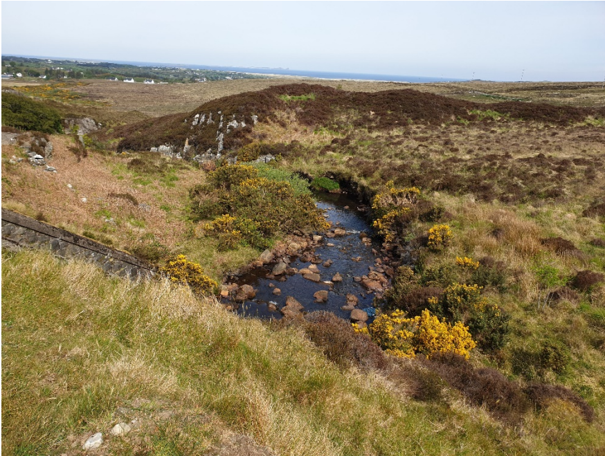
Bridge at crossing with Lough Agher stream (facing north).
